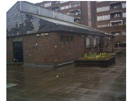
The old Community Hall will be demolished and a new one built.
